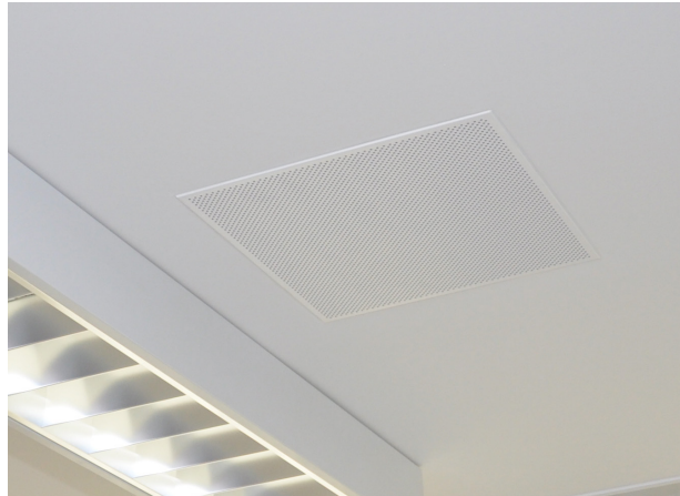
Fig. 7: Opticlean installed in a gypsum plasterboard ceiling
